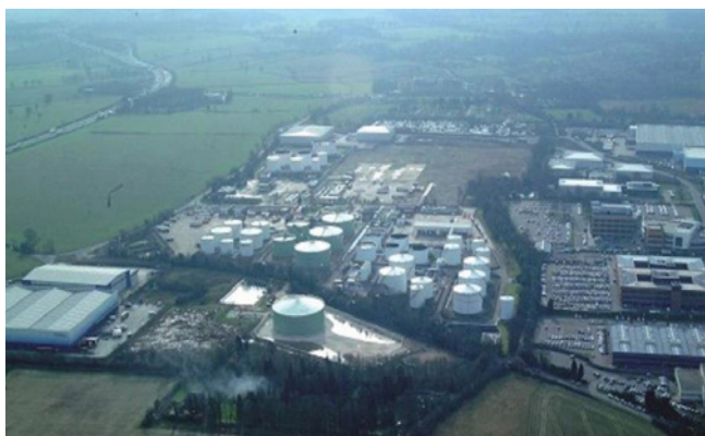
Figure 7: Buncefield Terminal Before Blast
