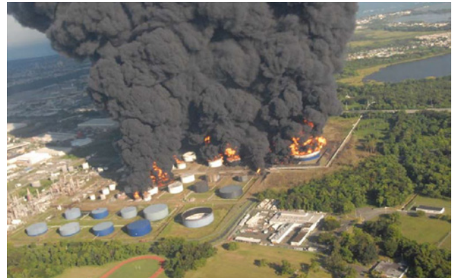
Figure 11: View of Terminal Day after Incident
