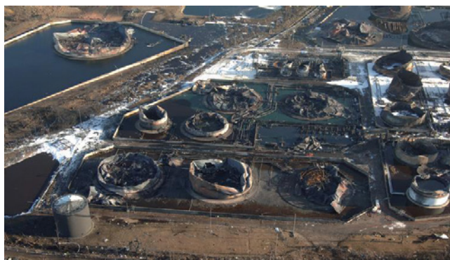
Figure 9: Buncefield after the Incident with the Culprit Tank T-912 Initiating Event at Center Foreground 6
