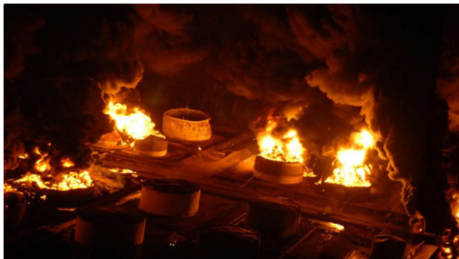
Figure 10: 2009 Capeco Tank Overflow Incident 7
